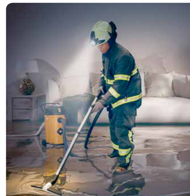
Rapid response to flooding or burst pipes.*
