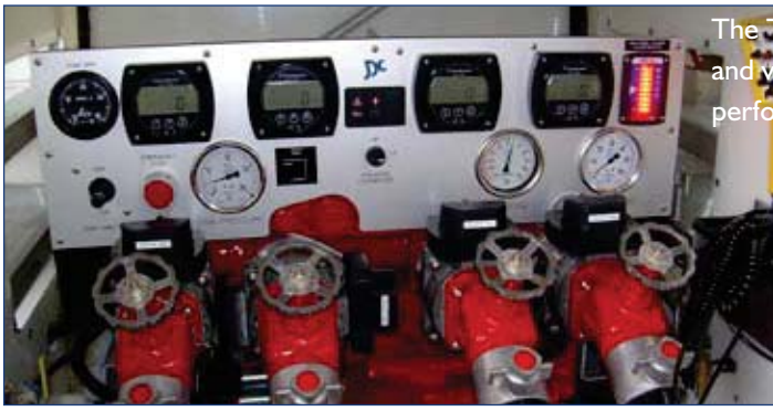
GMFRS Fire Service Year 2008 fire appliance pump bay.
